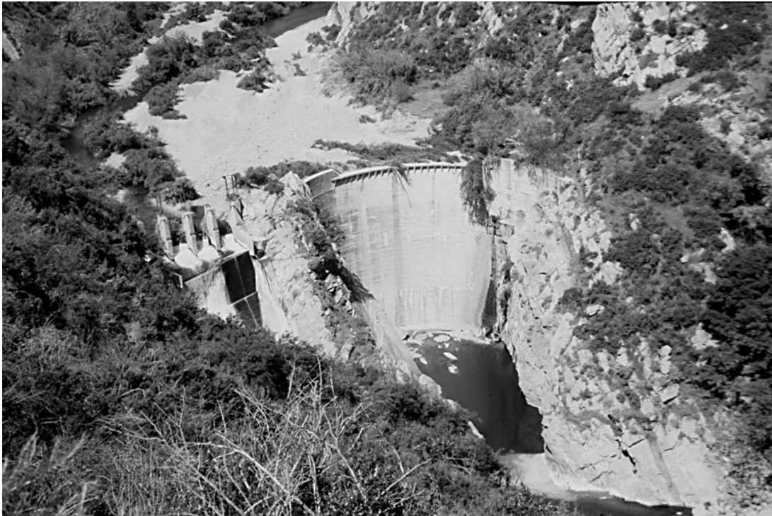
Figure 2. Rindge Dam, Malibu Creek. Note vegetation colonizing stored sediments behind dam.
