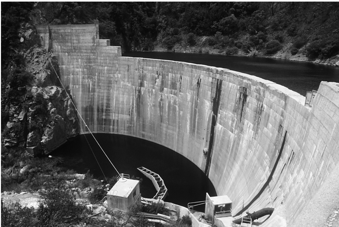
Figure 5. Matilija Dam. Note large notch removed from dam face, reducing storage capacity.
