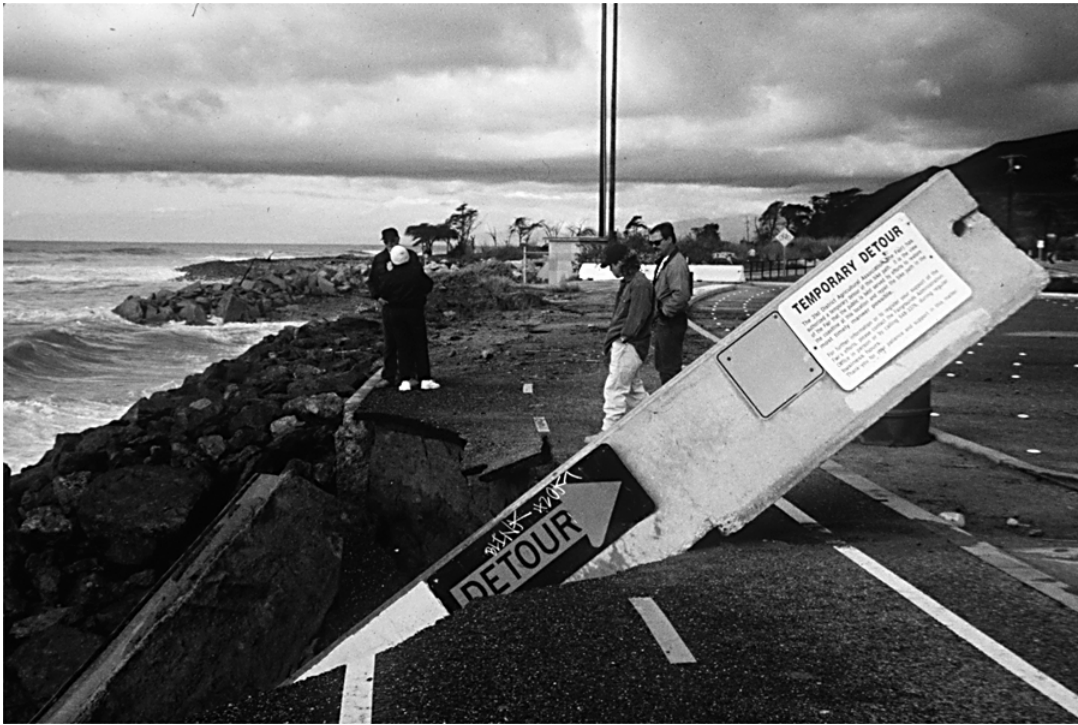
Figure 9. Damaged bikeway on Ventura River marine deltas due to coastal erosion induced by construction of dams in the Ventura River watershed.
