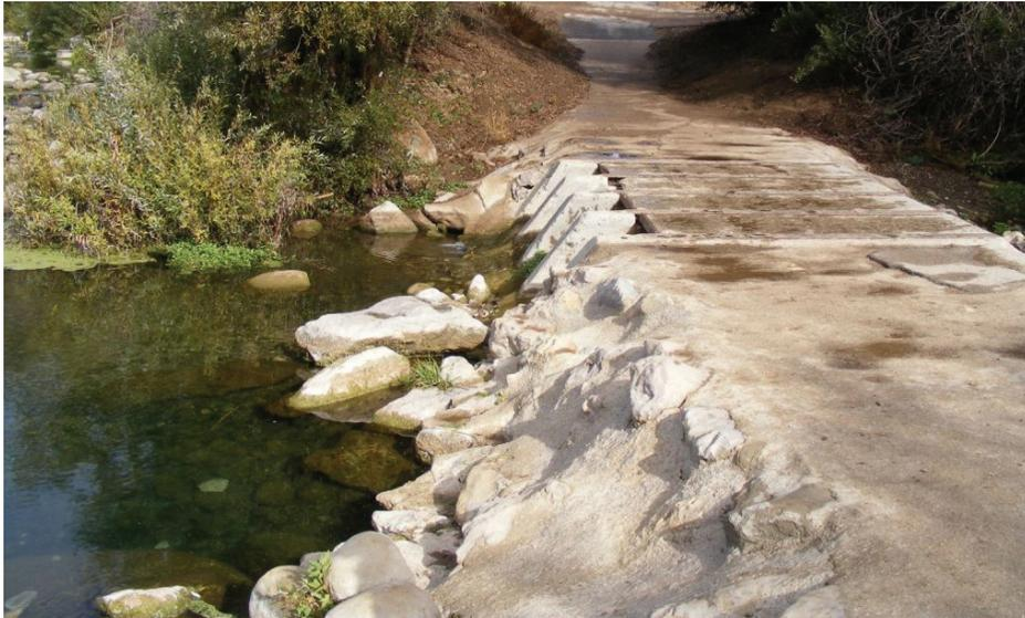
**Photograph 11:** Trail crossing, confluence of Ventura River and San Antonio Creek. It is designed to allow water to flow under the structure, minimizing scouring and down-cutting downstream from the structure.
