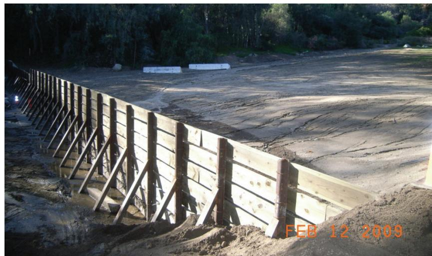
**Photograph 18:** A trash rack providing emergency protection to areas downstream (example from outside of the San Antonio Creek Watershed).
