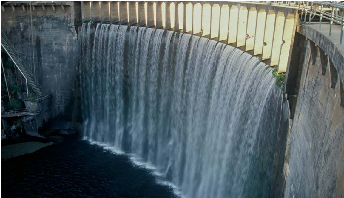
Figure 2. San Clemente Dam
