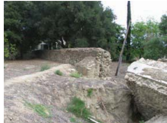
FIGURE 10.13 Historical aqueduct remnant undermined by erosion.
