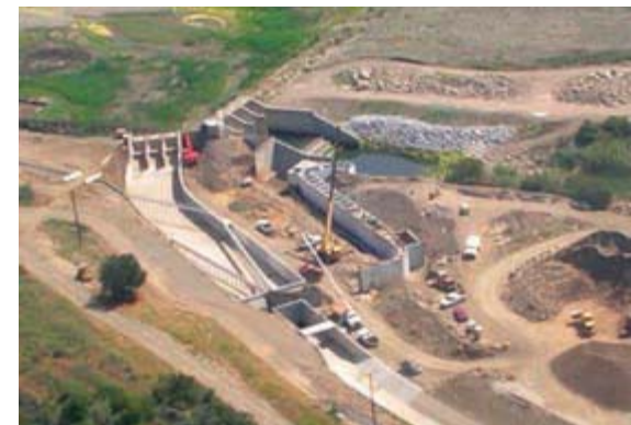
FIGURE 3.21 The Robles Diversion Dam removes up to 500 cubic feet per second of surface water from the Ventura River approximately eight miles upstream from the proposed parkway area. The canal to Casitas Lake can be seen leading from the diversion structure on the left. To the right of that diversion is a fish passage facility constructed in the mid-1990s. Photo: Greimann 2006.
