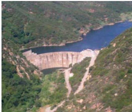
FIGURE 3.20 Matilija Dam, approximately ten miles upstream from the top of the proposed parkway area, holds back approximately 53% of the sediment that would otherwise flow in the Ventura River. Photo: Greimann 2006.
