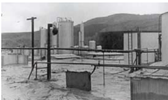
FIGURE 3.18. The 1938 flood was smaller than several events that have occurred during the past twenty years. However, it caused over one million dollars in damage (URS 2004) and inundated oil fields along Ventura Avenue. Nine years later, the Army Corps of Engineers completed construction of a levee to protect structures that intruded on the floodplain in this area and in the city of Ventura to the south. Photos: Museum of Ventura County; Ventura County Star.
